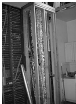
Space around Ducts may be a path
